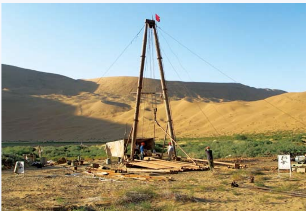
Hydrogeological drilling in a desert area
